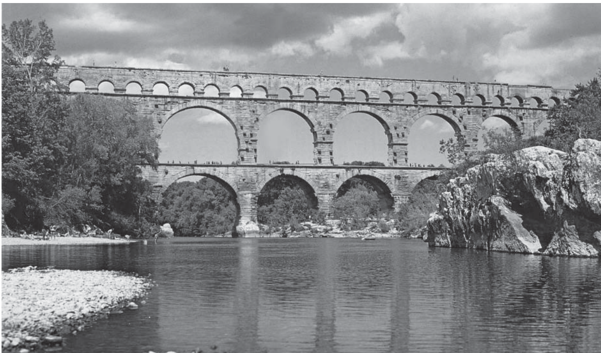
Pont Du Gard, built more than 2,000 years ago, the highest aqueduct built by the Romans. We will see this extraordinary feat of engineering from around the year 19 B.C.
